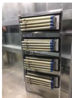
AtmosAir 508FC systems in Discharge of AHU
